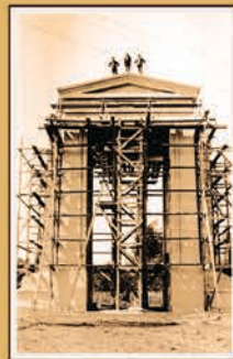
Construction of the Peace Arch 1920.
